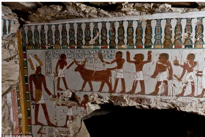
Figure 21.19 Collapsed ceiling and severely damaged wall section
